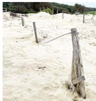
Sand fences have not been maintained
